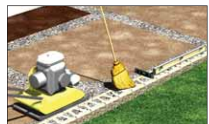
Backfill behind and in blocks, level and compact. Sweep top of blocks.
