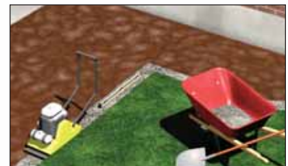
Install wall rock, level and compact.
