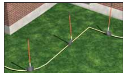
Layout and mark wall location.
