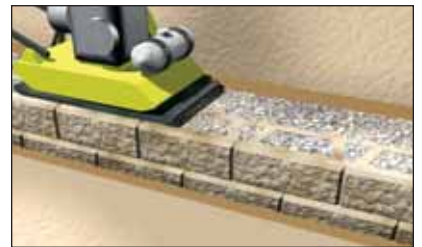
Backfill and compact.
