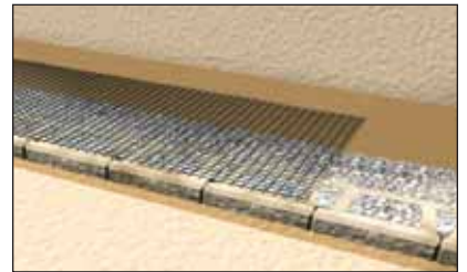
Install AB Grid Reinforcement if needed.
