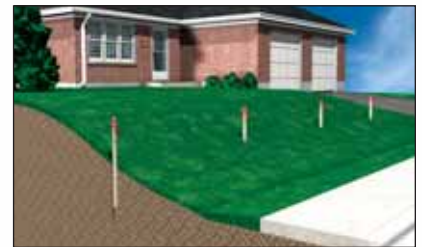
Layout and mark wall location.
